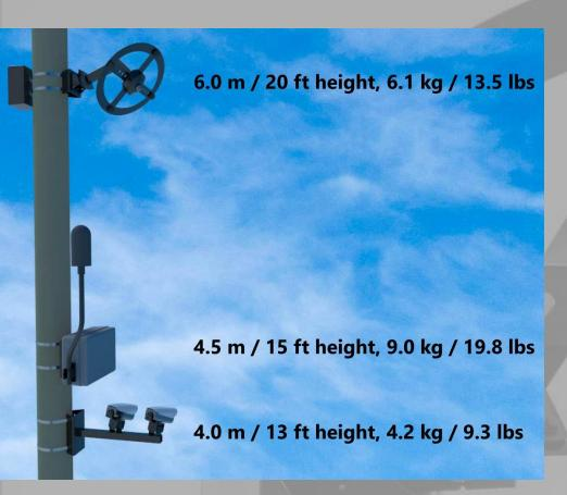
$SoundVue^{TM}$  is frequently installed on street lamp columns as we find that they are located in the right position relative to the road and are a cost effective alternative to constructing a new, bespoke powered pole.
